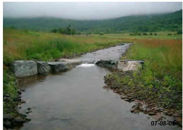
Figure 3.19 Rock Cross-Vane
