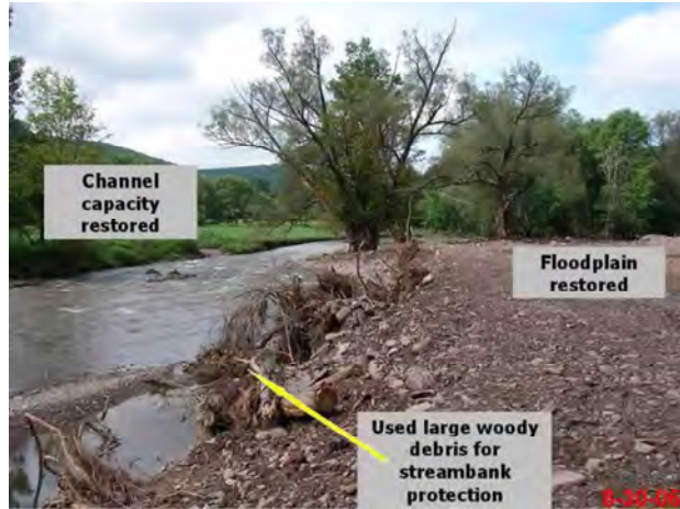
Figure 3.18 Stream construction using Regional Bank full Hydraulic Geometry values, typical cross-section and root wad.
