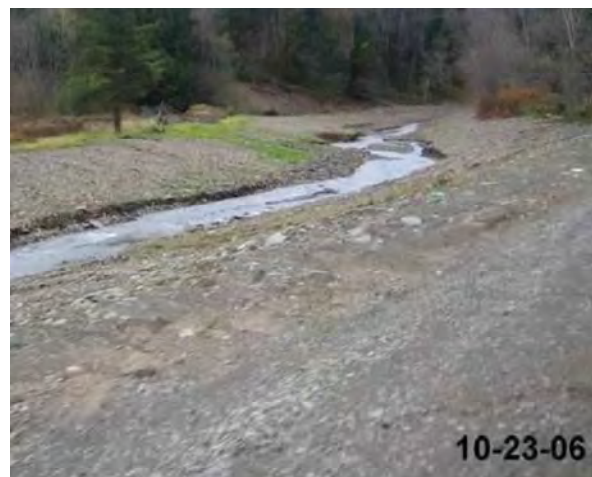
Figure 3.3 Two months of stream channel evolution.
