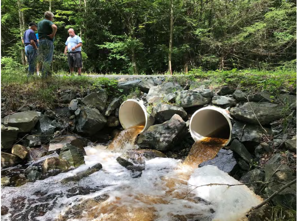
Figure 16. Outlets of twin 36-inch culverts on Potter Creek at Fifty Six Road, approximately one mile upstream of Campfire Girls Dam
