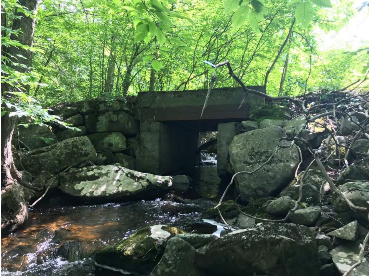
Figure 6. Looking upstream at relic culvert from a disused road crossing of the Quacken Kill tributary between Route 2 and Roark Road
