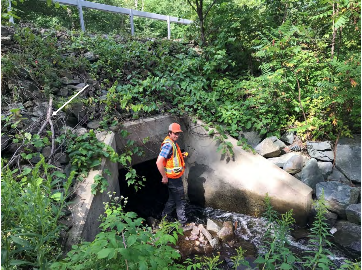
Figure 5. Tributary culvert entrance beneath Route 2 near intersection with Stuffie Street in Grafton. Note concrete repairs to wingwalls and headwall and rip rap repair to right bank. White arrow indicates debris most likely deposited during a recent high flow event when flow backed up behind the culvert.
