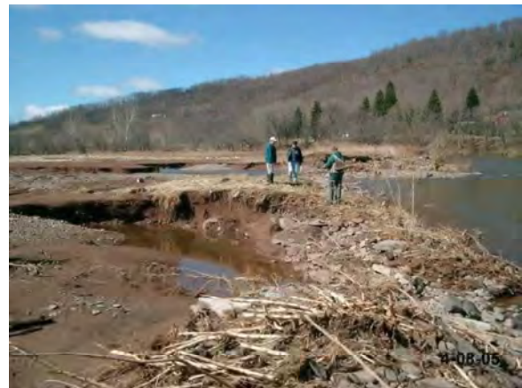
Figure 3.12 Berm that was breached in 2005 storm event
