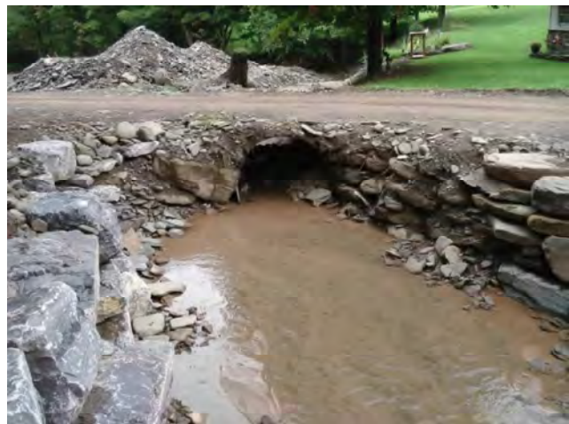
Figure 2.17 Culvert Conveying on Holliday Brook Colchester, NY
