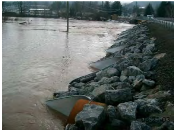
Figure 2.19 Floodplain culverts along Delaware County Route 2 Hamden, NY
