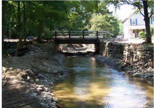
Figure 2.18 Bridge results in elimination of Floodplain
